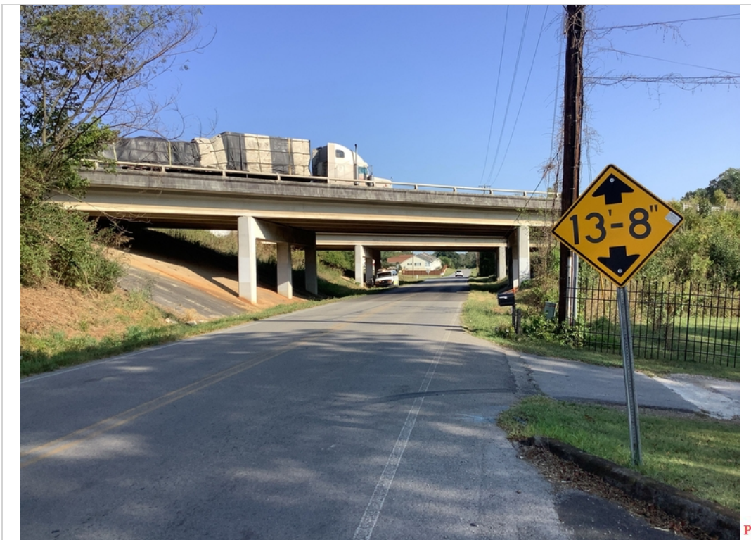
Underpass forward clearance sign
