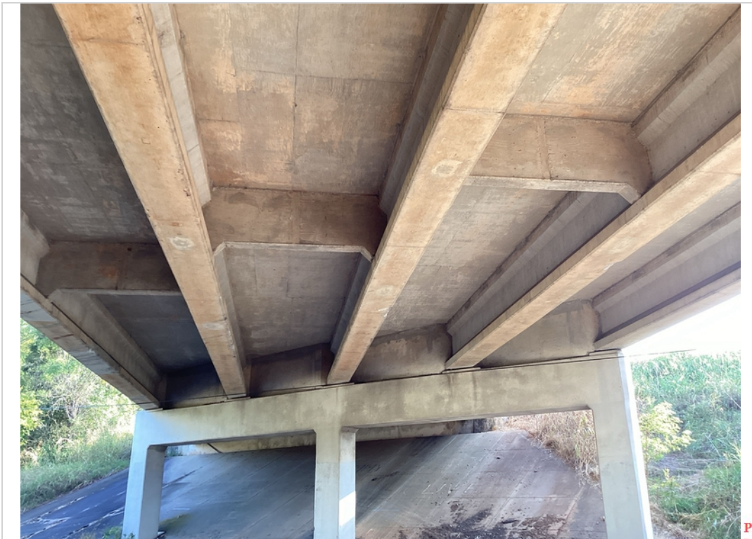
Span 2 - View underneath
