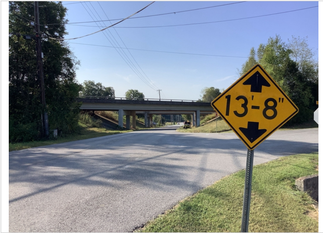
Underpass back clearance sign
